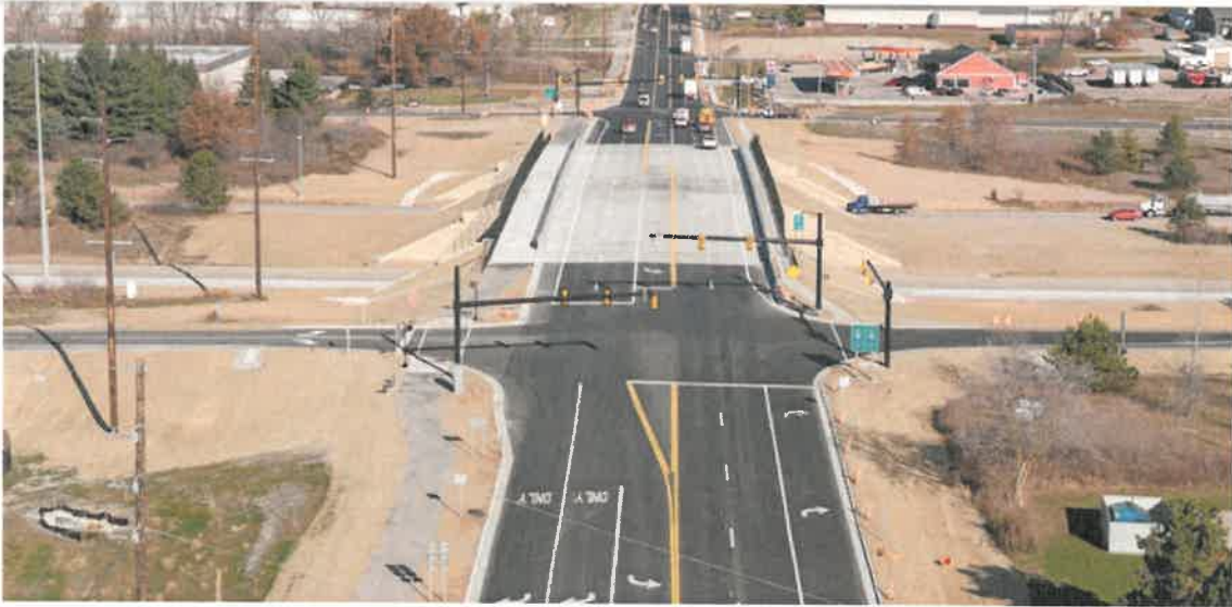
Photo of the Fruit Ridge Avenue Bridge. Image provided courtesy of MDOT photography unit.
